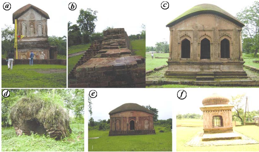
Figure 5. Historical temples in Silchar (South Assam) region. Note extensive ruins of the Khaspur king's ward ( b ) and two temples ( a and d ) at Taligram. Due to restoration work at other two temples ( c , e and f ), damage assessment is not possible. f , Singhdwar, note the extensive tilt. The observed tilt in ( a ) and ( f ) appears to be due to local site affects.
