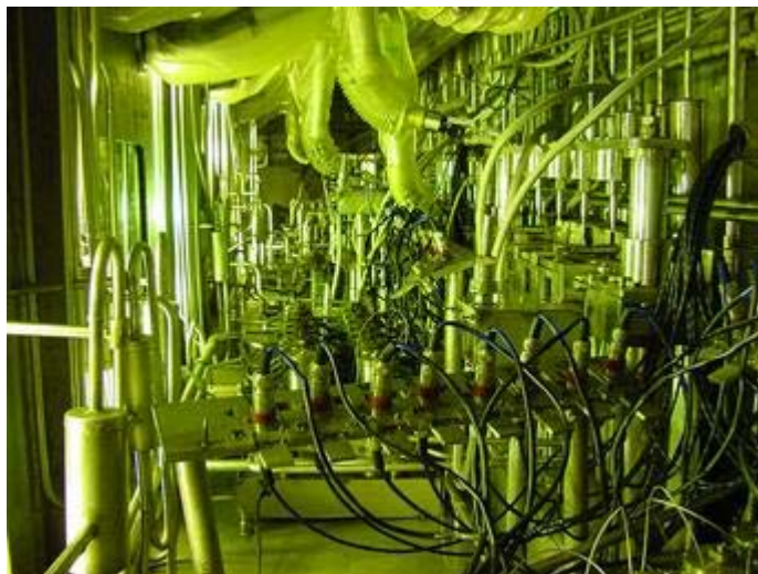
The compact hot cell facility for FBTR spent fuel reprocessing was commissioned in 2003
