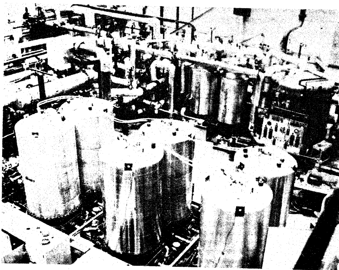
Figure 4. 1 MW fuel cell plant built under the TARGET-Program.
