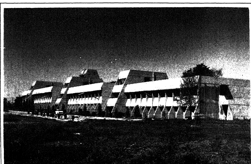
The institute's main building.
