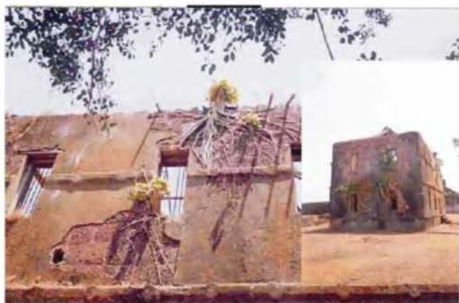
Figure 3. Main house at Jaigad, Ratnagiri District ( 17^{\circ}17'45.15''\text{N} , 73^{\circ}13'38.57''\text{E} ). Different Ficus species such as Fa attached to the same building. The roots could have at best helped displace the decomposing plaster. Inset, the lateral view: the trees penetrating through broken windows.
