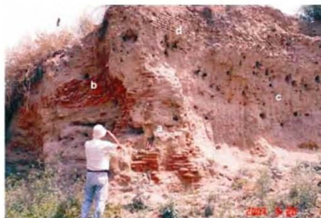
Figure 3. Eastern part of the main outcrop on south side of the road. Settlement I: a, the lower level with large red baked bricks and mud bricks with sand. b, Distorted red bricks. Settlement-II: c, In the upper level remain of tilted wall with rubble of bricks and sand, small size bricks. d, Dirty-white, unstratified, sand-silt containing pottery and bone fragments and red bricks.
