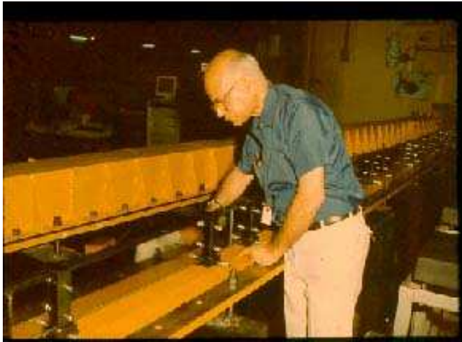
Figure 2. Neutron guides under installation at Dhruva reactor.
