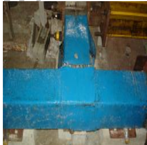
(d) Embedded additional reinforcement and confined with CFRP sheets
