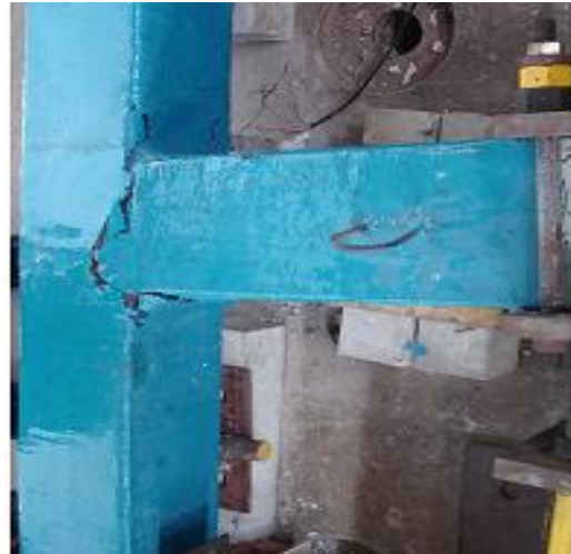
(b) CFRP laminate and confined with CFRP sheet
