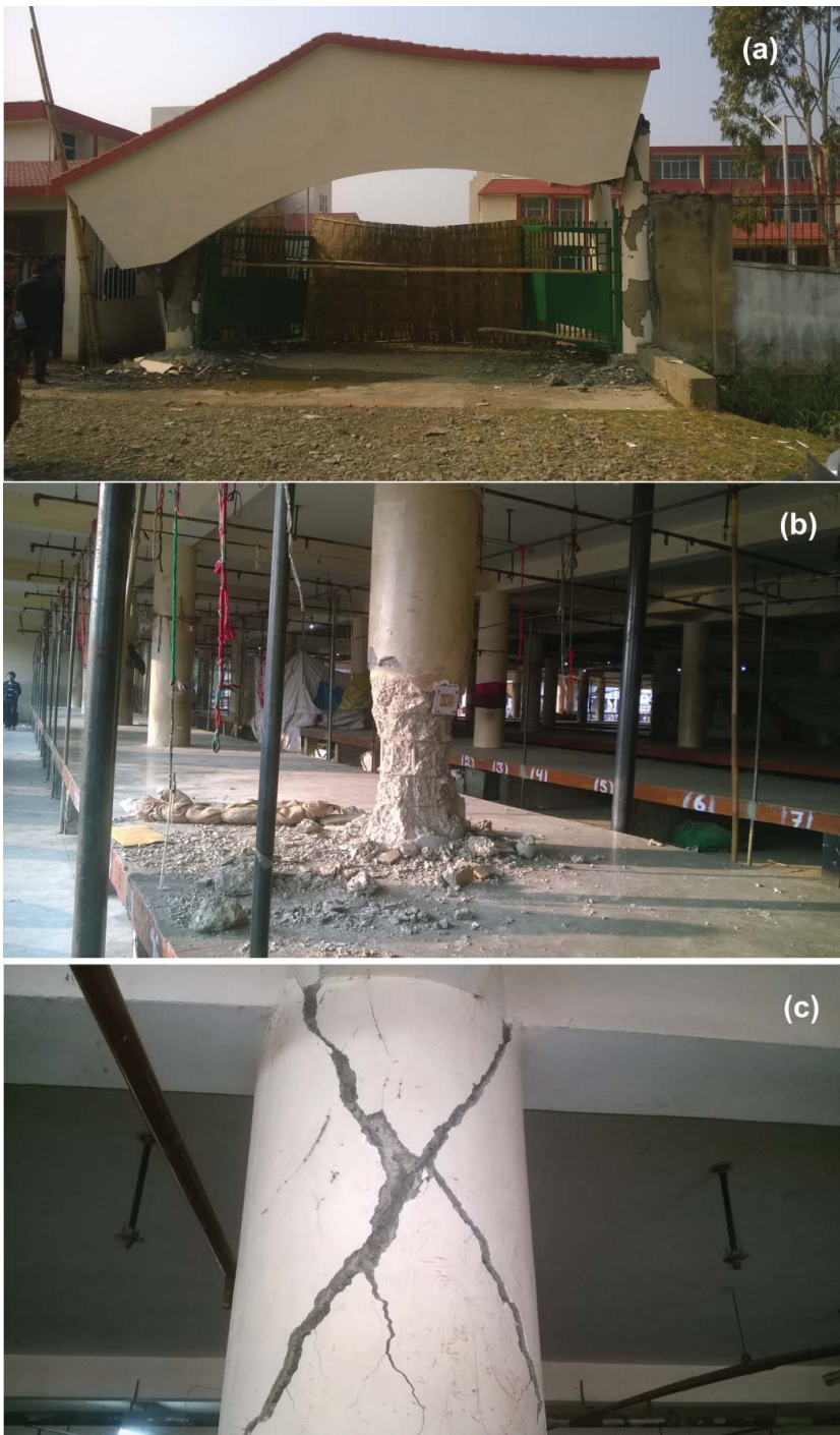
Figure 4. Photographs showing damage in Imphal: (a) Agricultural University gate, (b) and (c) damage to the pillars of Ima women market through crushing and shear cracks.
